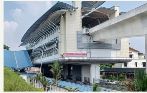
USJ 21 LRT Station
